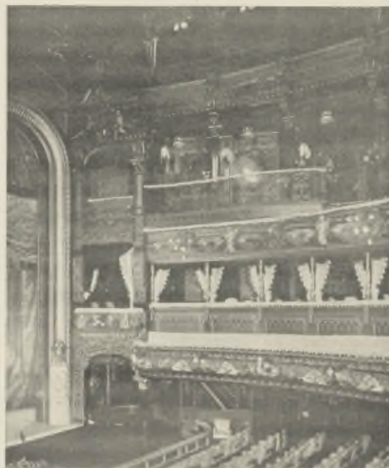
"EMPIRE" VARIETY THEATRE, LONDON. VIEW OF AUDITORIUM.
