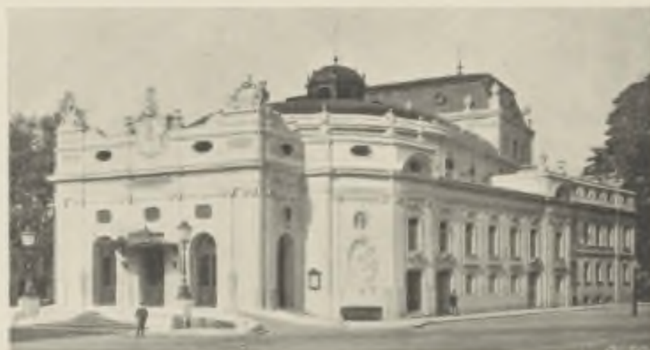
MUNICIPAL THEATRE, SALZBURG. GENERAL VIEW.
