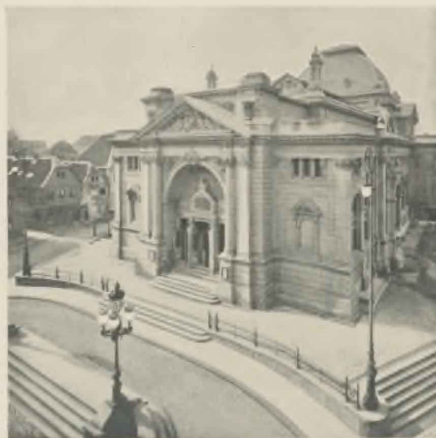
MUNICIPAL THEATRE, ESSEN. GENERAL VIEW.
