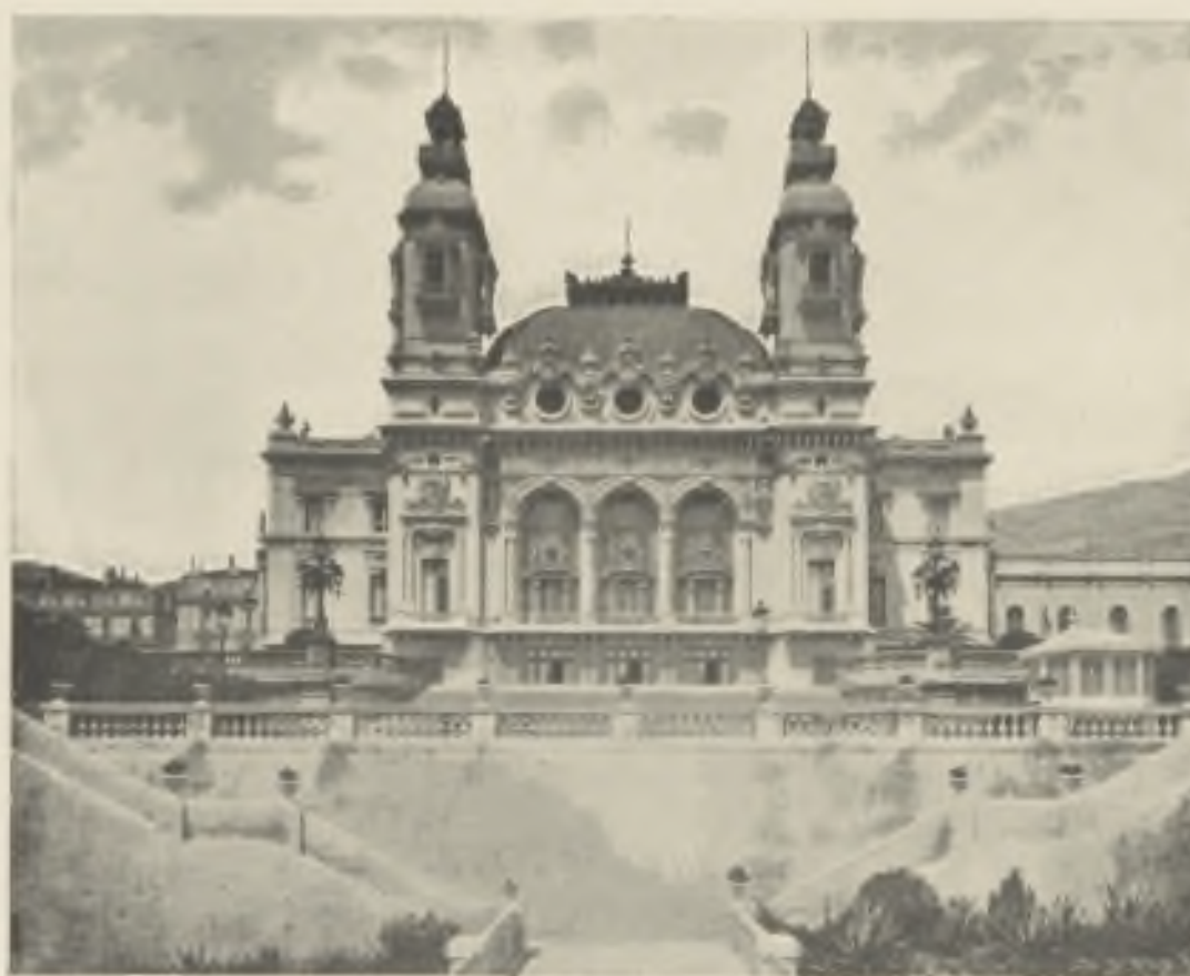
CASINO THEATRE, MONTE CARLO. GENERAL VIEW.
