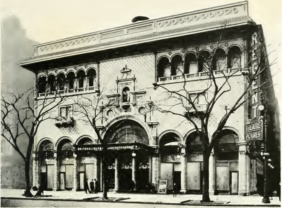
VI. REGENT THEATRE, 116TH ST. AND SEVENTH AVE., NEW YORK CITY Thomas W. Lamb, Architect
